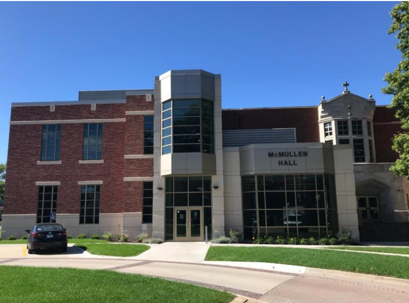
Entryway to McMullen Hall, where most conference events occur this week. McMullen Hall underwent an extensive renovation, reopening in summer 2020 with more than 37,000 square feet of space.
